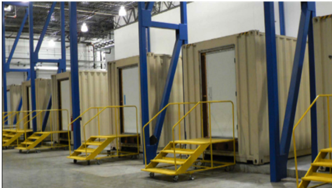
Figure 4.15: Google's container-based datacenter.
